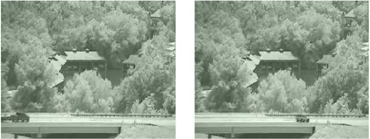
Figure 6.7: Sample Frames from Video Sequence of a bridge from a side-view perspective (Source: Aimetis).
